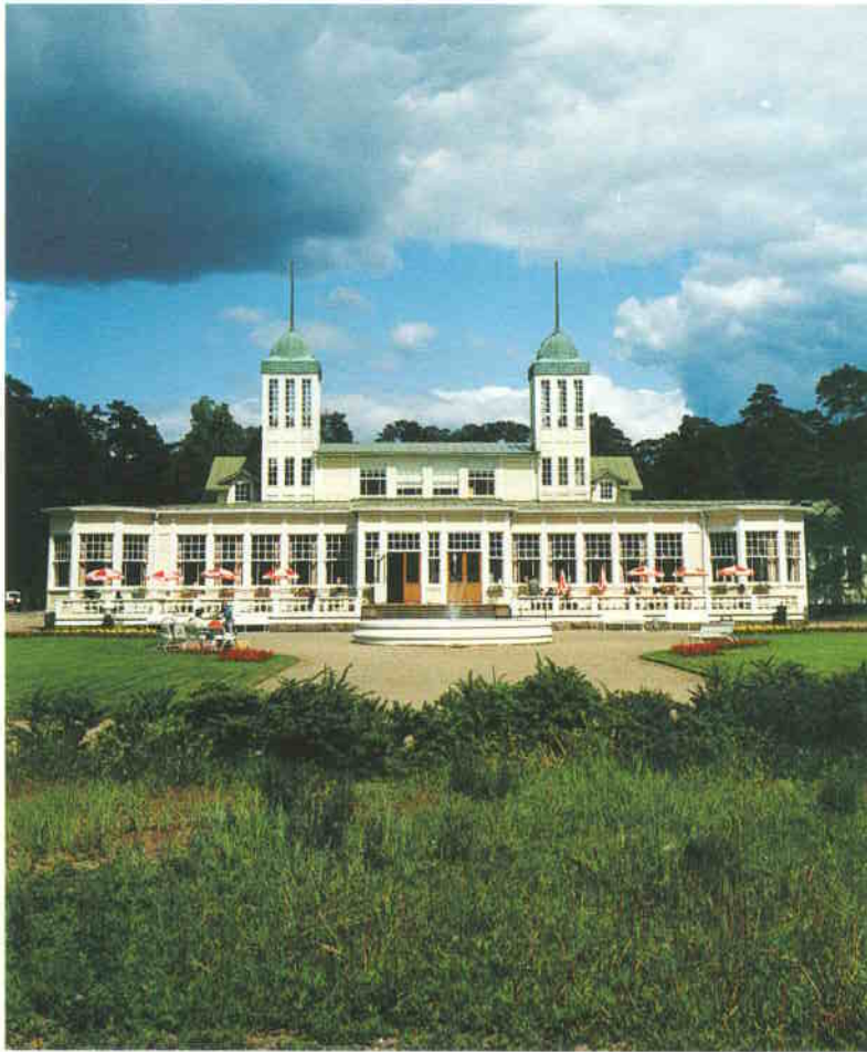
Casino of a small southcoast town Hanko (founded 1874). The repairs of the building were financed by grants from the Ministry of the Environment.
