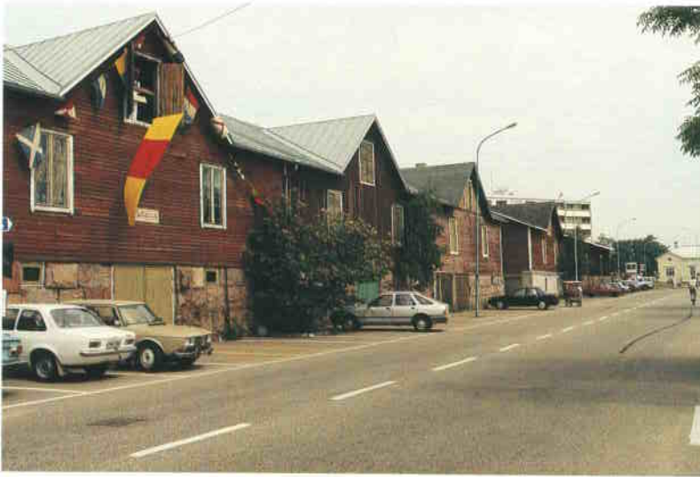
The Hanko harbour storage buildings will be repaired with a grant from the Ministry of the Environment.
